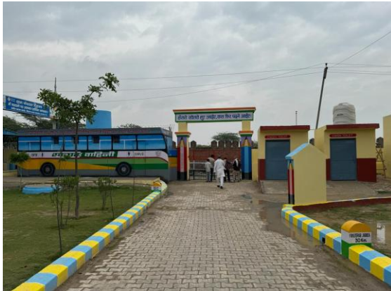
After — new main gate and toilet blocks
