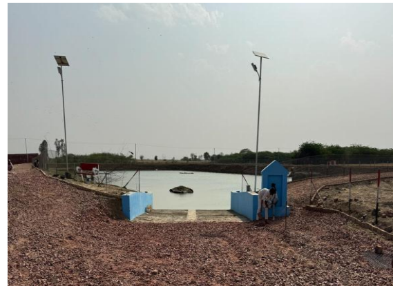
Completed pond — ramp, solar lights, fencing, benches
