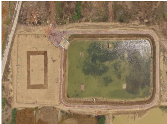
Aerial view — completed pond
