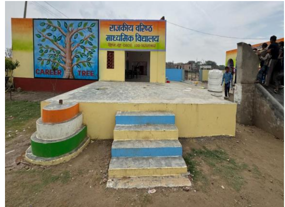
After — refurbished classrooms and corridor
