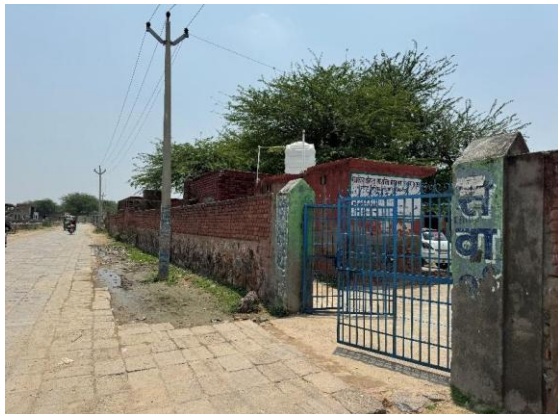
School campus before — dilapidated kitchen block
