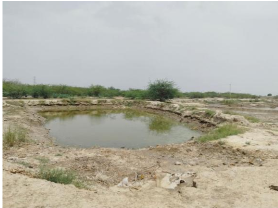
Pond — dry and heavily silted before work
