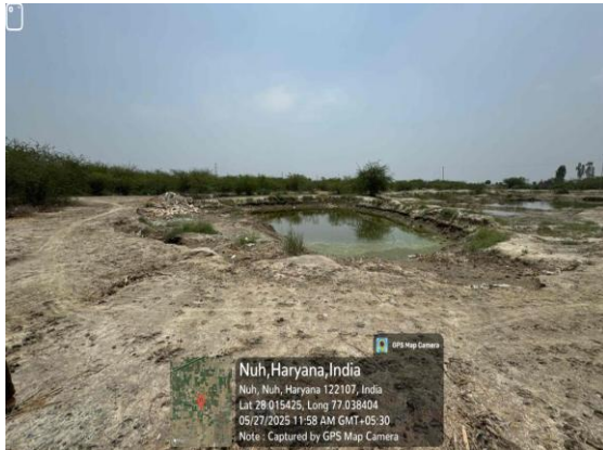
Pond silted and non-functional
